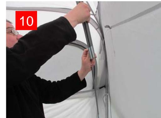
Carefully assemble the pole by inserting each pole section into the adjoining ferrule.
